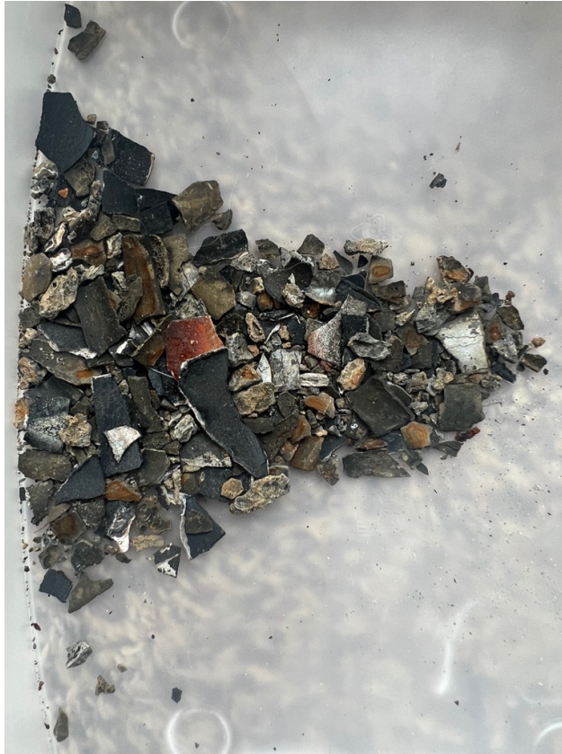
Large metal particles flushed from the heat pump
