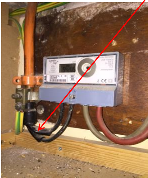
Example of VIR covered conductors
